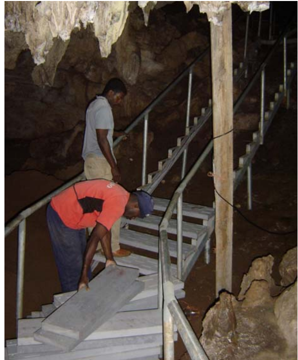
Planking is placed on the first stair - the heavier, non-slip plank type
